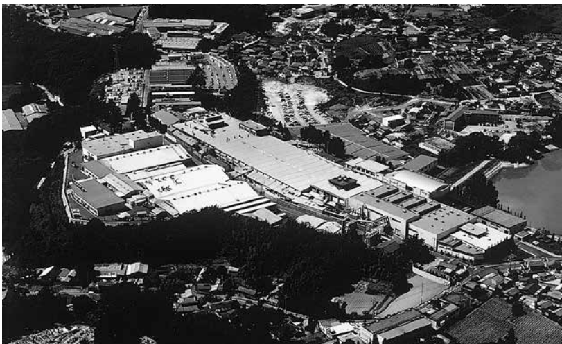
KITZ Nagasaka Plant, Japan
